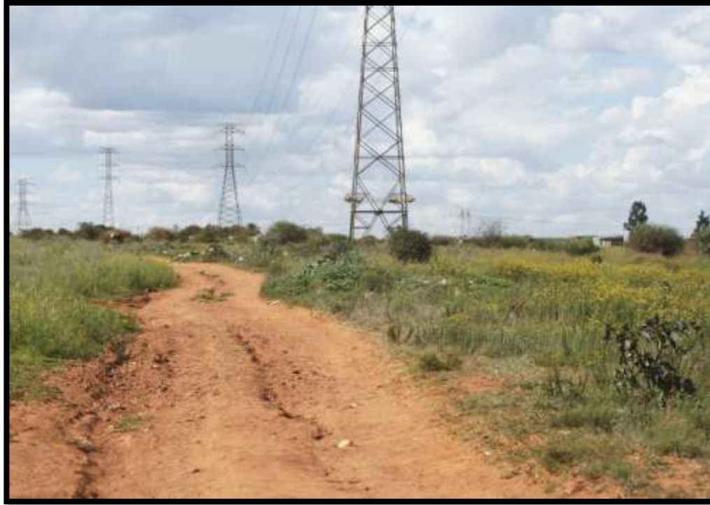
Photograph 6. Pylons and informal roads run through the site
