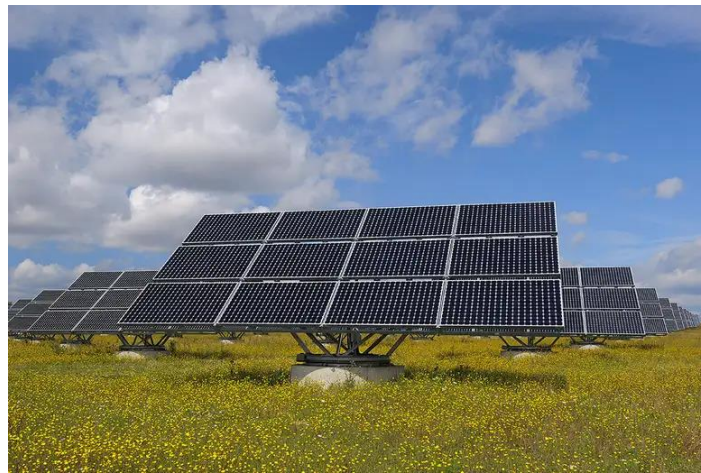
Figure 2.6: An Example of a double-sided solar panels that track the sun (New Scientists-2020)
