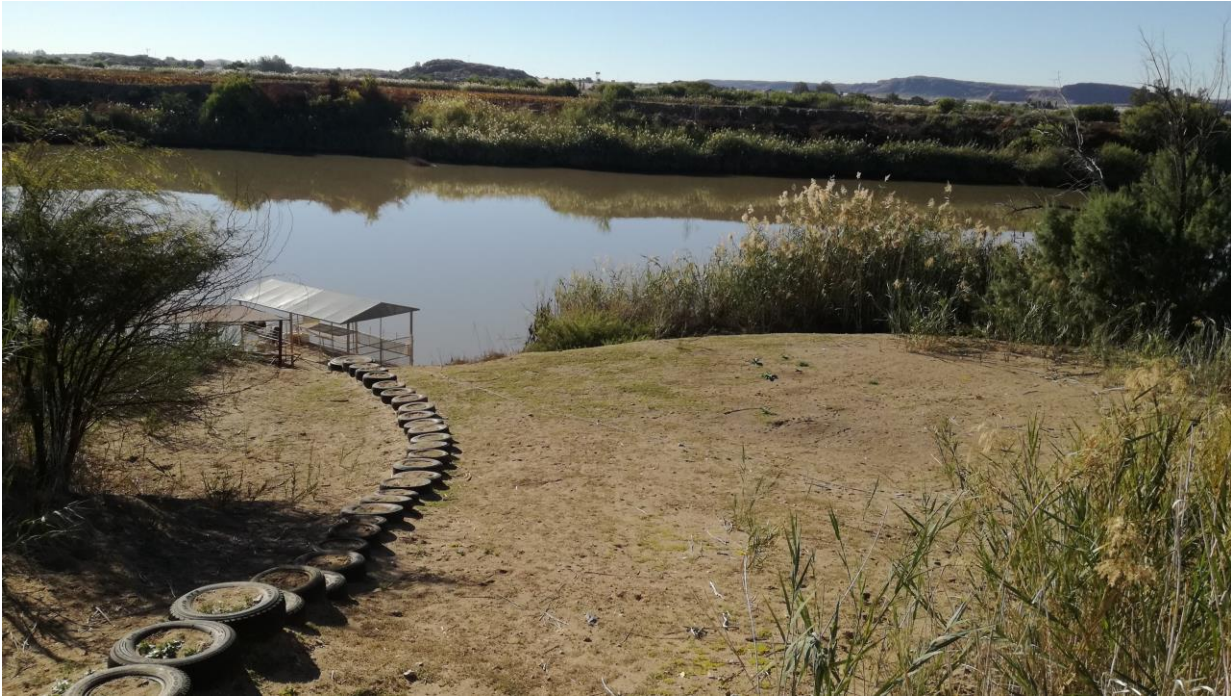
Figure 4: General view of the proposed pumpstation site on the banks of the Orange River. Note existing pumpstations.
