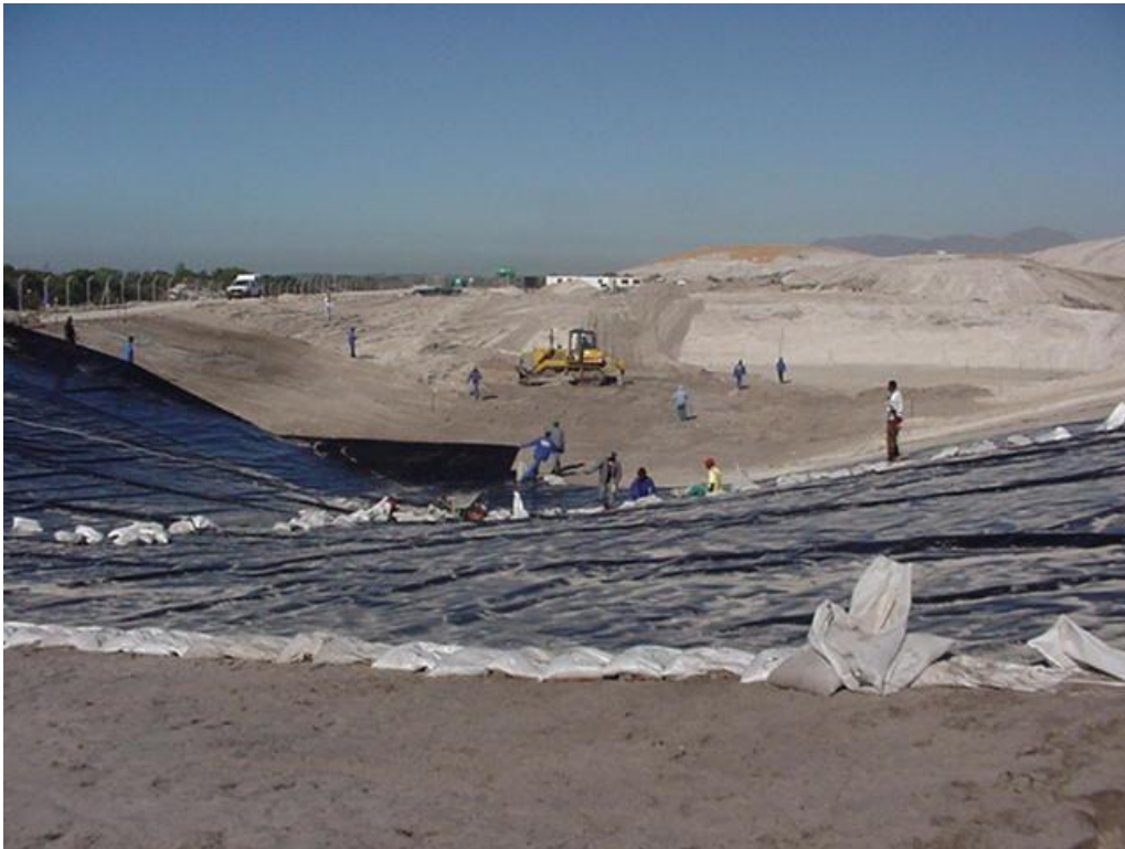
Figure 2-3: Example of the typical waste cell construction
