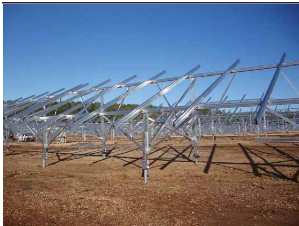
Figure 4.4 Typical Anodized Aluminium Frame
