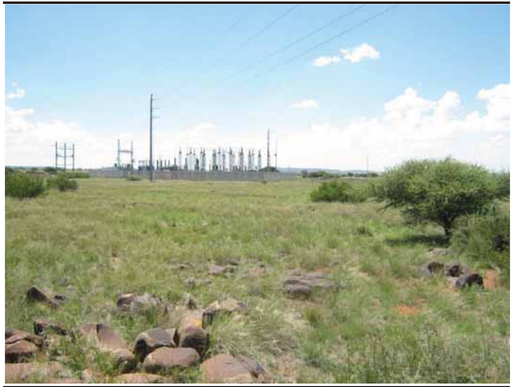
Figure 5.15 View of site, looking north, showing existing 132kV transmission line and substation
