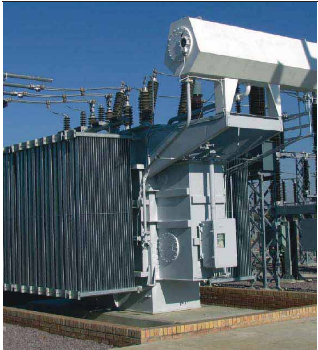
Figure 4.9 Power Transformer
