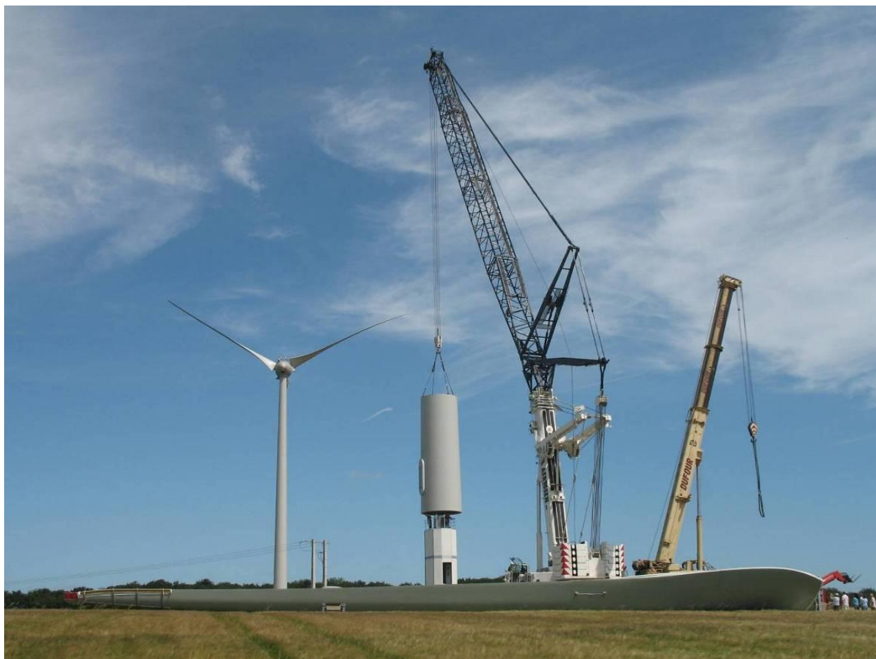
Plate 2-4: Assembly and erection of the tower sections
