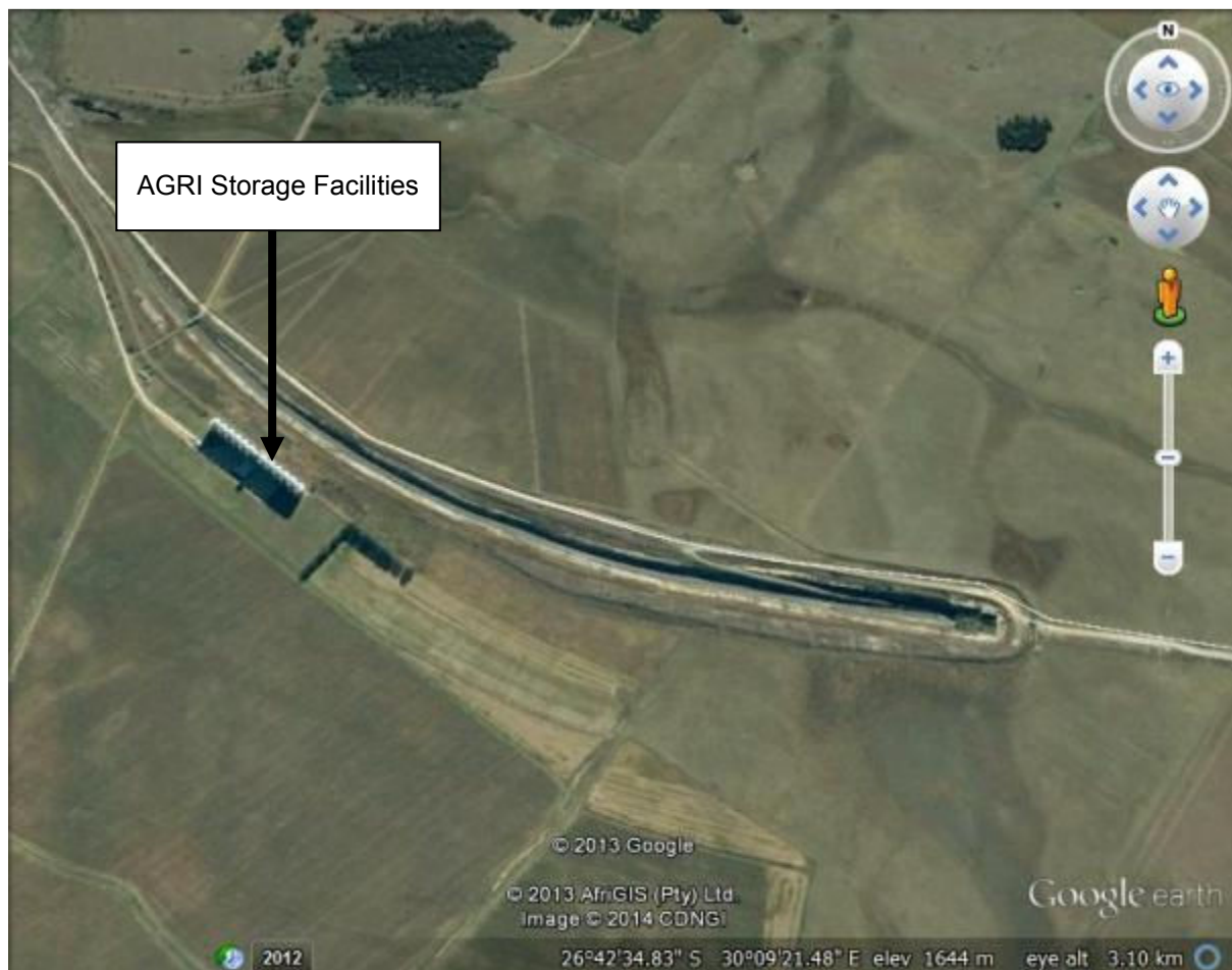
Figure 22: View of the AFGRI storage facilities to the western tunnel exit
