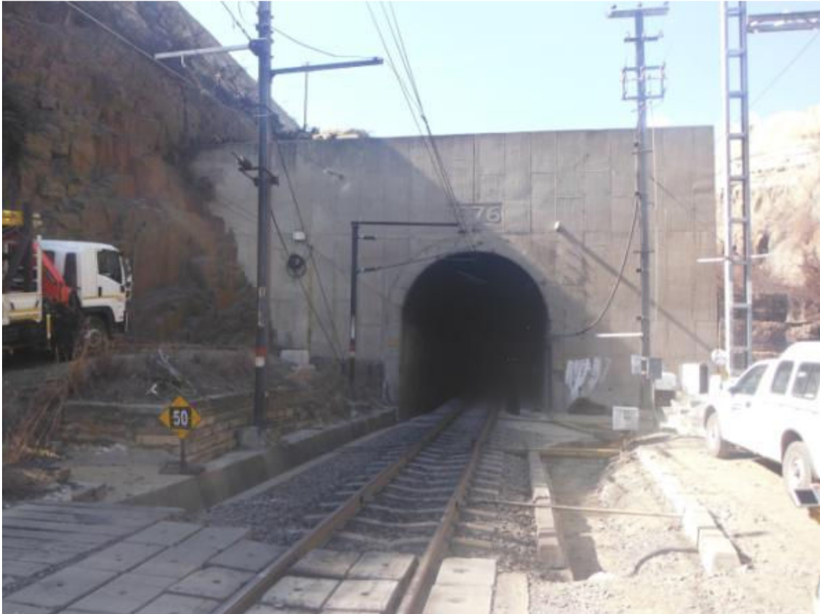
Figure 5: Representative view of the existing tunnel.
