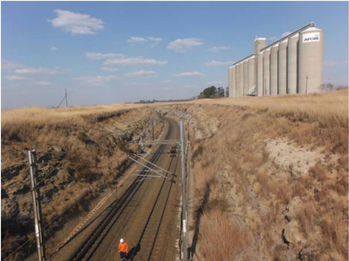
Figure 15: View of AFGRI storage facilities and the Richards Bay Coal Line section towards the north of the proposed project site.
