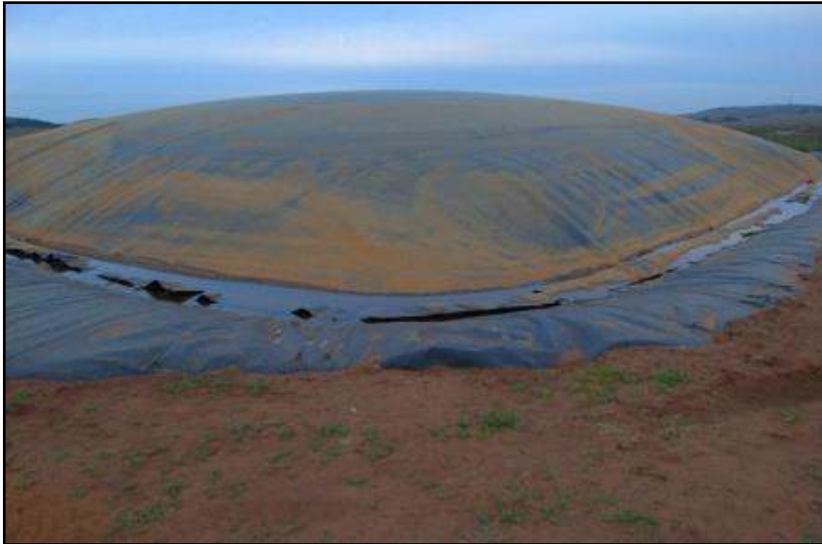
Plate 8: Example of a 'digester' covering an effluent dam.
