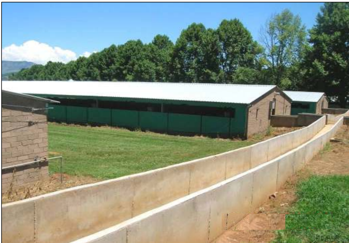
Plate 7: Concrete walkways for efficient control of pigs outside of houses.
