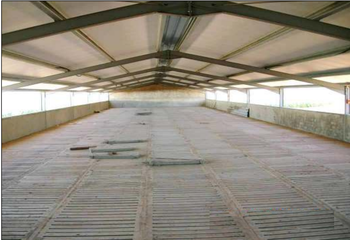
Plate 5: Proposed design showing slatted concrete floor.
