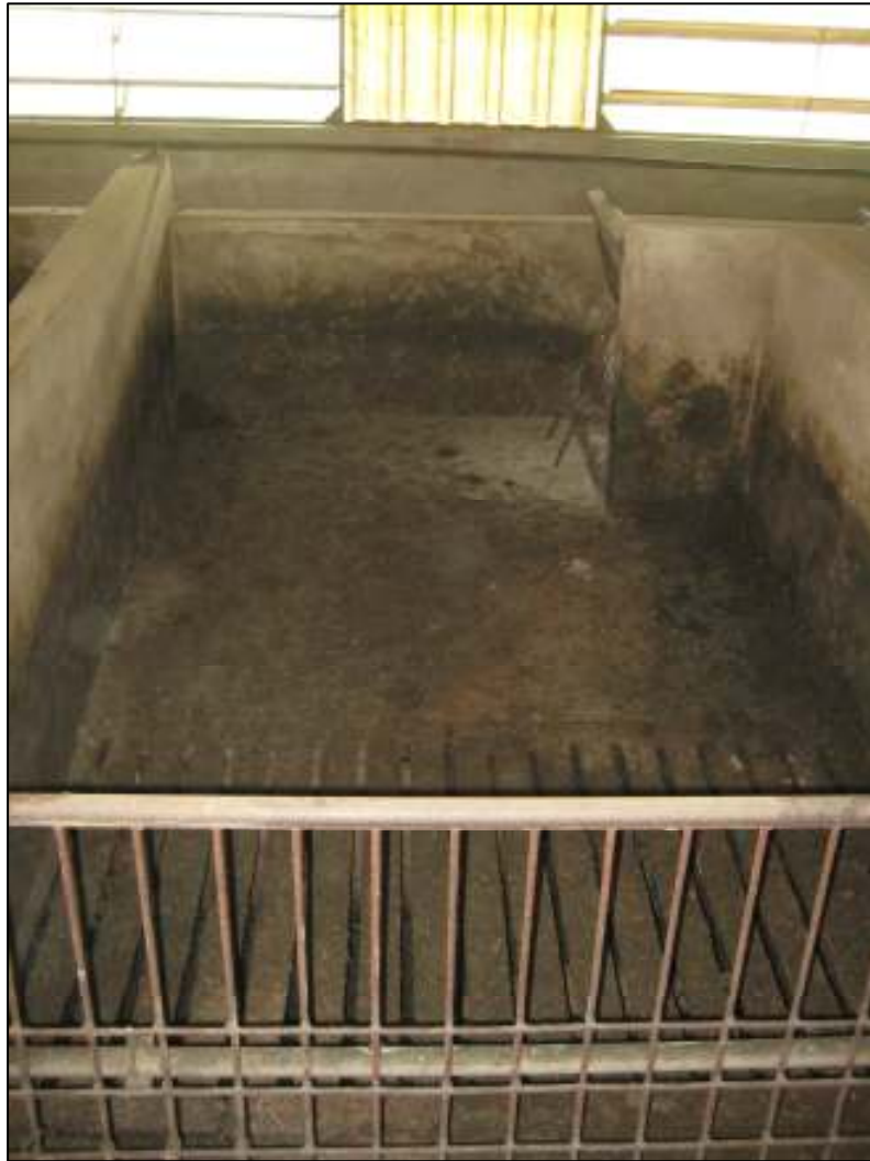
Plate 4: Existing piggery showing solid floors which result in dirty conditions and need high volumes of water for cleaning.
