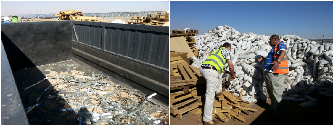
Figure 12 (a & b): Metal waste and saw dust and wooden pallets will also be a waste product that will require storage for recycling. Saw dust bags are used inside the boxes of panels during shipping to protect the solar panels. Wooden pallets (seen in figure above) are used to secure the products.
