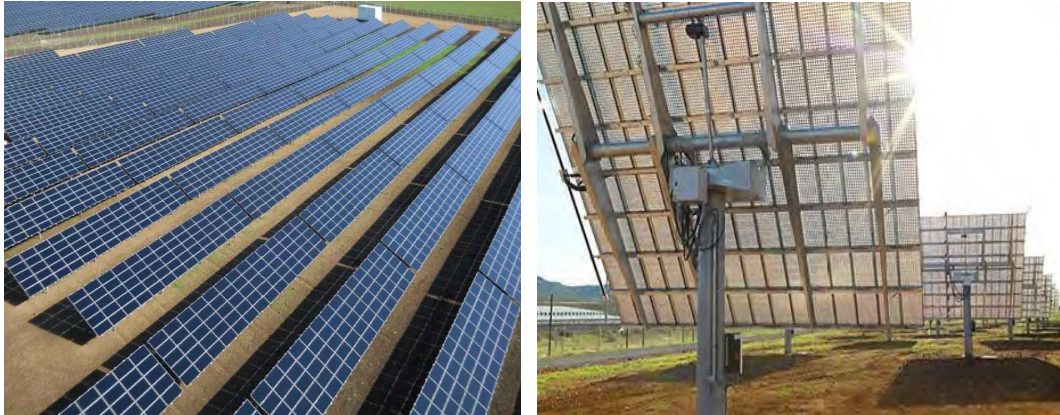
Figure 14 (a & b): An Example (from different sites) of a Photovoltaic Solar Farm (PV) – Double Axis Tracking System on Right (free standing panel installation), Single Axis Tracking System (five row table installation) on Left.
