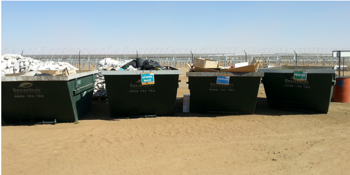
Figure 11: It is proposed to separate waste at source (to be recycled) and store it on site as per the image above that shows general waste, cardboard and plastic storage skips.
