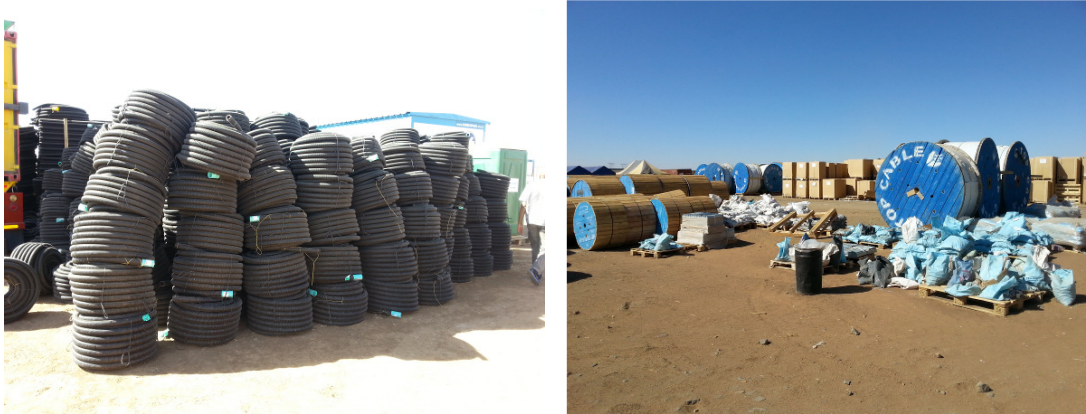
Figure 10 (a & b): An example of the kind of plastic tubing for the cabling that is proposed to be stored and another example of a material storage area (figure B).
