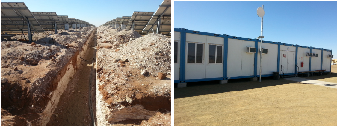
Figure 7 (a & b): The figure on the left shows the proposed cable trenching and the figure on the right shows the types of temporary offices proposed.
