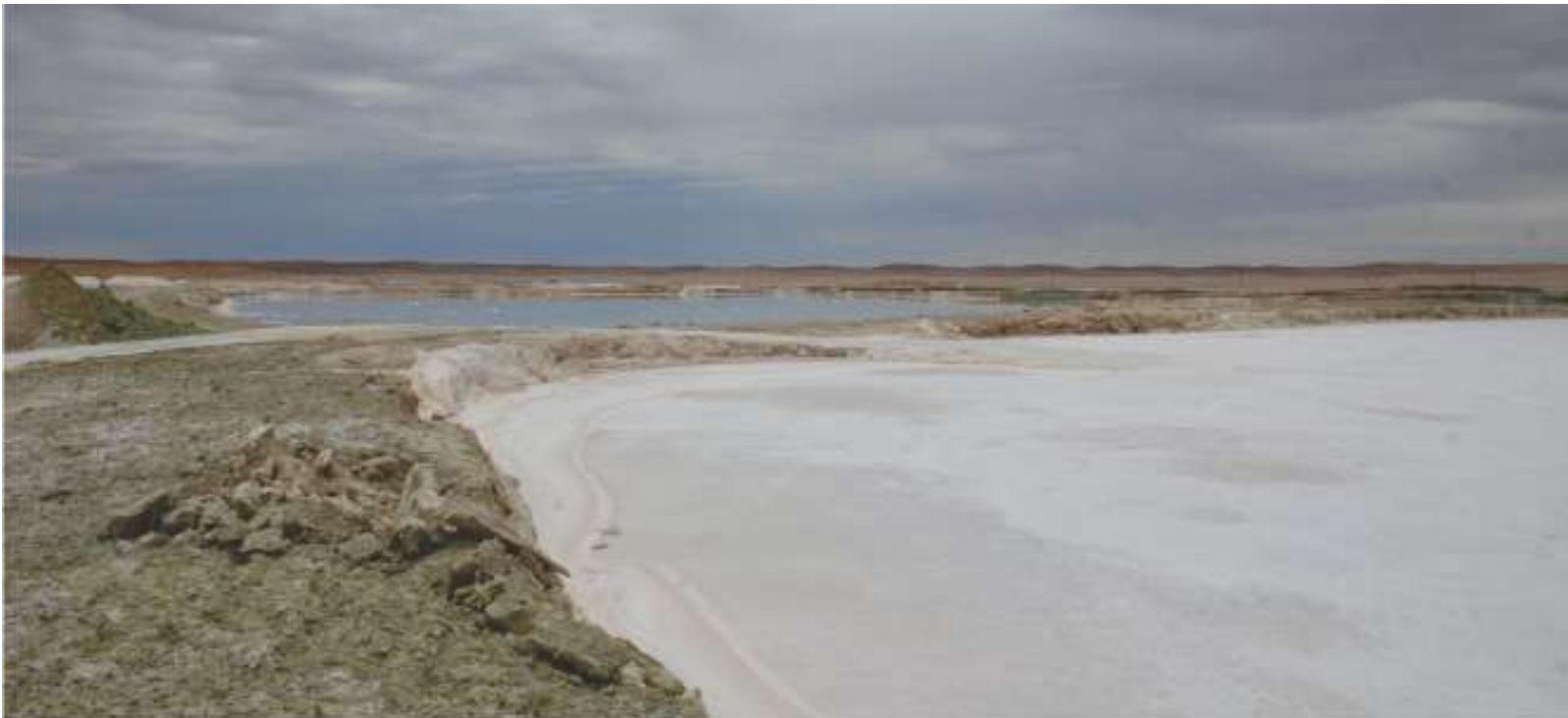
Photo 6: Photo shows a concentration pond in the background and an evaporation pond almost ready for harvesting in the foreground typically found at solar salt mines on pans in the area.
