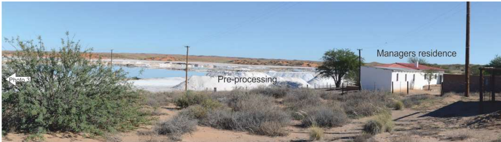
Photo 4: Looking north and west from Generator house showing overall view of operations
