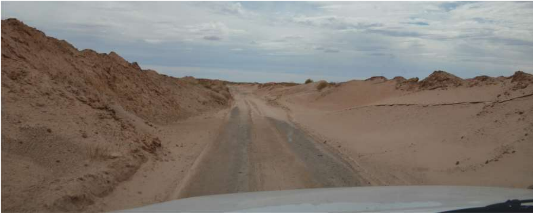
Photo 10: The status of the access road. Maintenance and sand control measures are required
