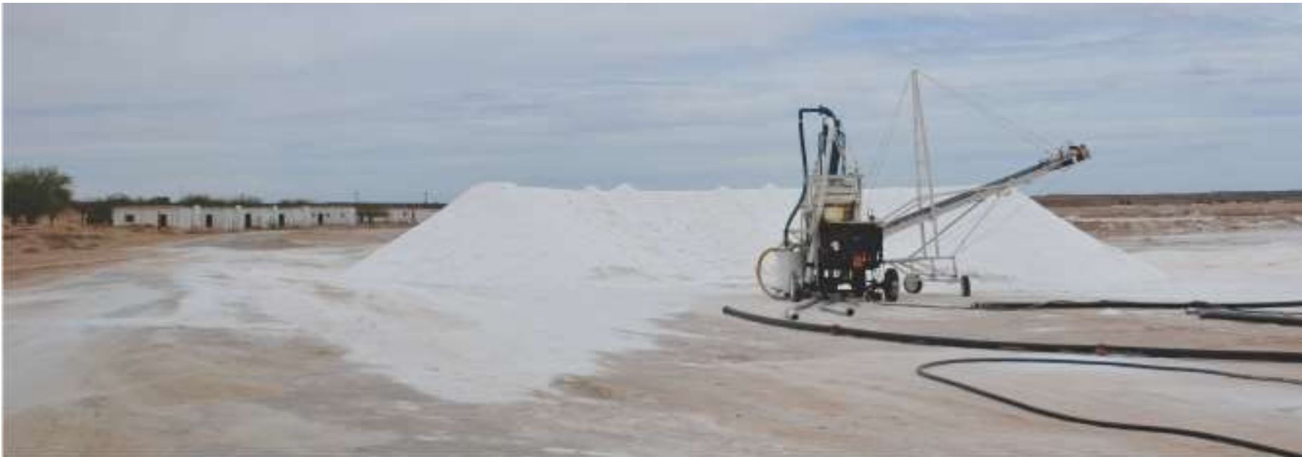
Photo 8: The last stage in the processing is the final sorting through a cyclone with material fed to roving conveyor. The whole machine is on wheels which allows it to move back to generate an elongated clean salt stockpile with loading form the other end. The waste water from this process is fed to a holding dam /small evaporation pond as per photo 9 below.
