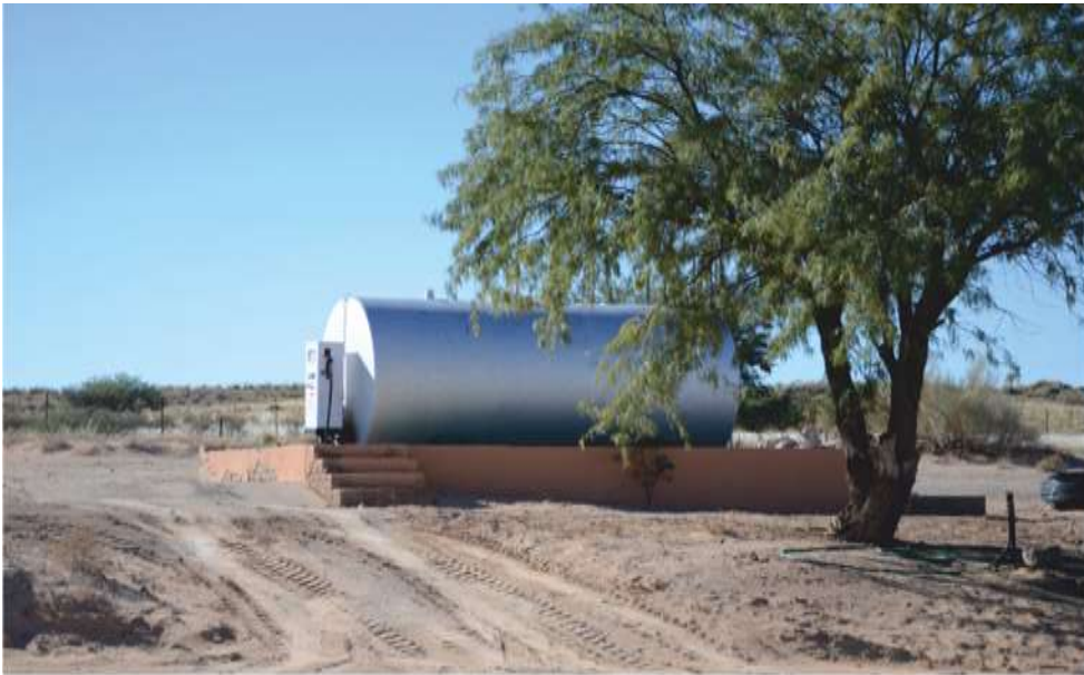
Photo 2: Main diesel tank left (23kl) and Generator house and 2kl diesel tank (photo right)
