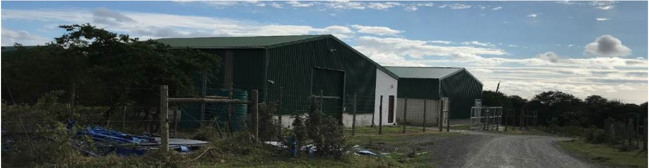
Figure 10: Existing access road, workshop area and storage sheds on the site
