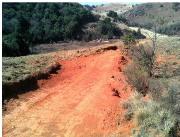
Figure 25: Road to be stabilised by surface cross drain (intervention W42C-02-213-00) looking in a south-easterly direction
