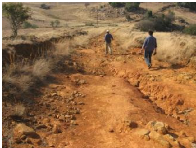
Figure 20: Old road requiring closure and rehabilitation (Intervention W42C-02-208-00)
