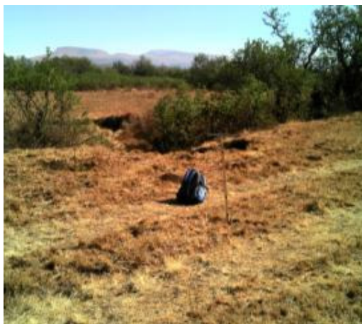
Figure 15: Earthen diversion berm, W42C-01-208-00 looking in a north-westerly direction
