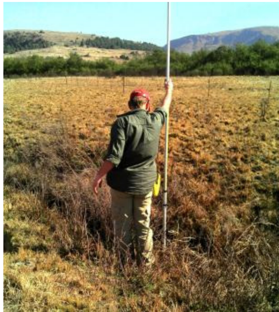
Figure 10: Earthen diversion berm, W42C-01-204-00 looking in a south-westerly direction
