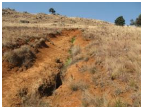
Figure 28: Deactivation of erosion gully next to road (W42C-02-216-00) looking south-southeast
