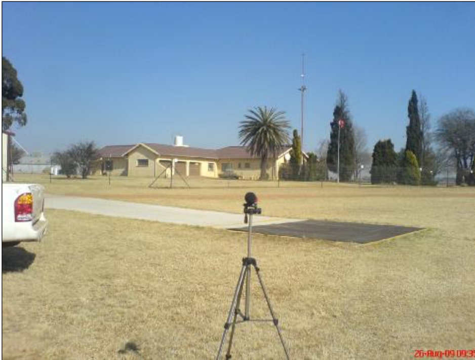
Figure 1: View of the residence on portion 39 of the farm Middelbult 235 IR
