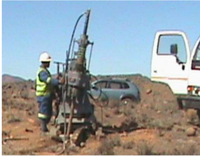
Photo 6: Scale of core drilling equipment to be used on site
