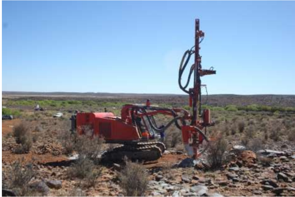
Photo 4: Percussion drill rig to be employed
