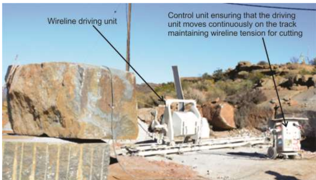
Photo 9: Typical wire line cutting
