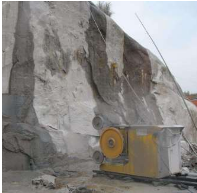
Photo 8: Typical wire line cutting
