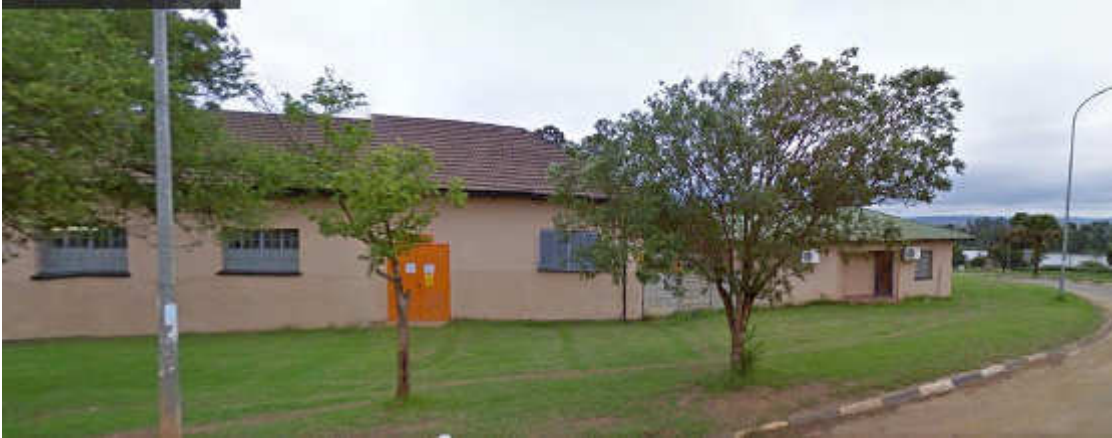
Figure 6: Brand Street view (north western corner), structures older than 60 years
