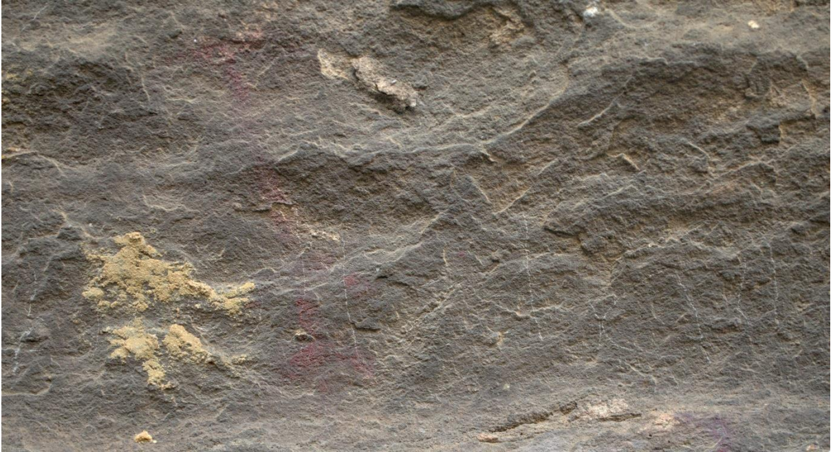
Figure 12: Dust and graffiti on the panel of 9d, covering some of the images.
