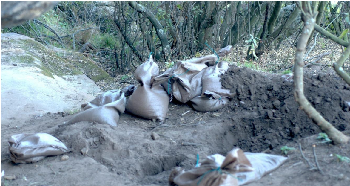
Figure 14: Possibly disturbed excavation or left without backfill.
