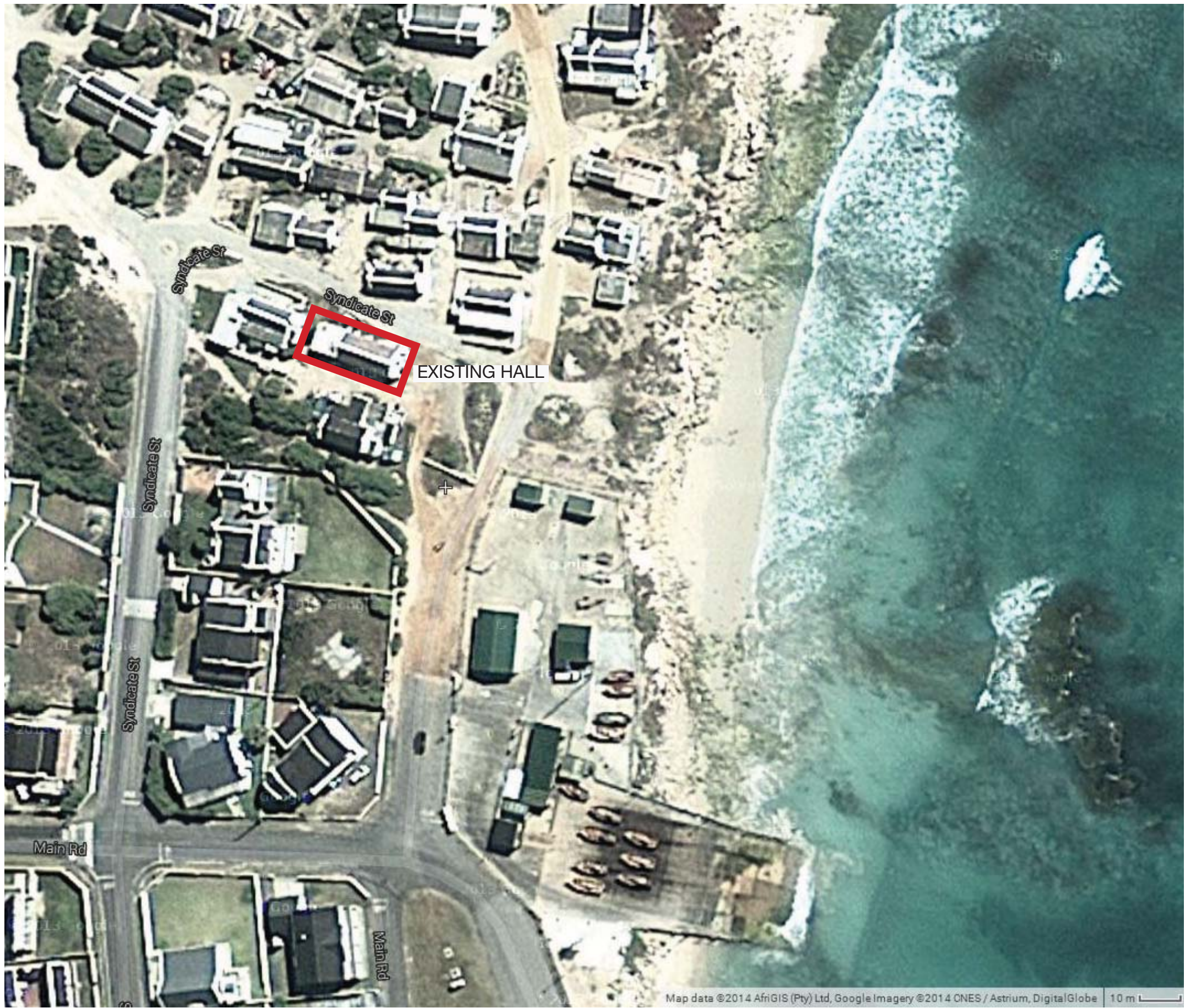
Google Earth aerial view of existing Fisherman's Union Hall in context
