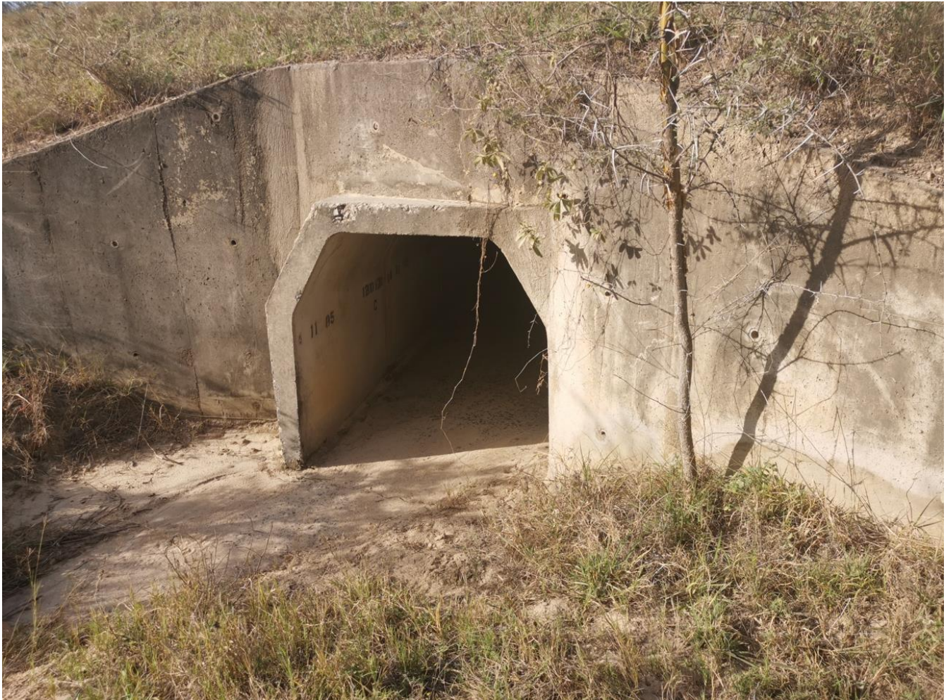
Figure 7 Stream C1 culvert 1200mm high x 1200mm wide
