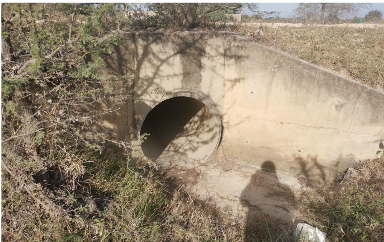
Figure 10 Stream C2 culvert 900mm diameter
