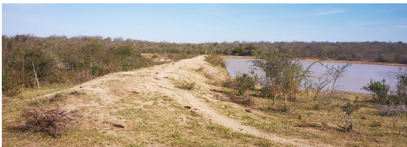
Figure 14 Stream C13 onsite
