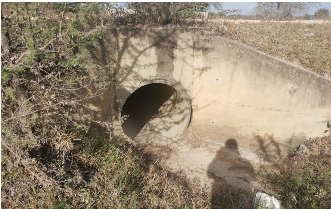
Figure 10 Stream C2 culvert 900mm diameter
