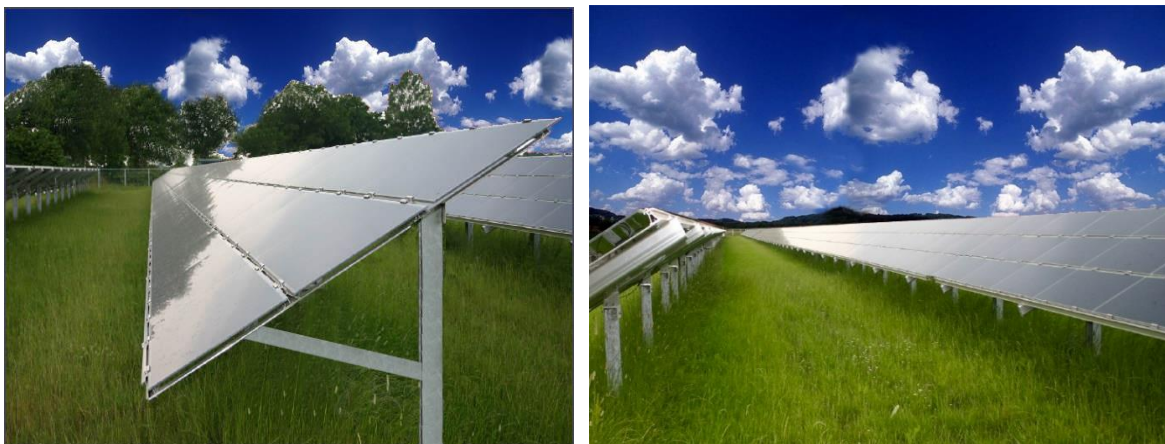
Figure 3. Lateral views of PV arrays mounted on fixed mounting systems
