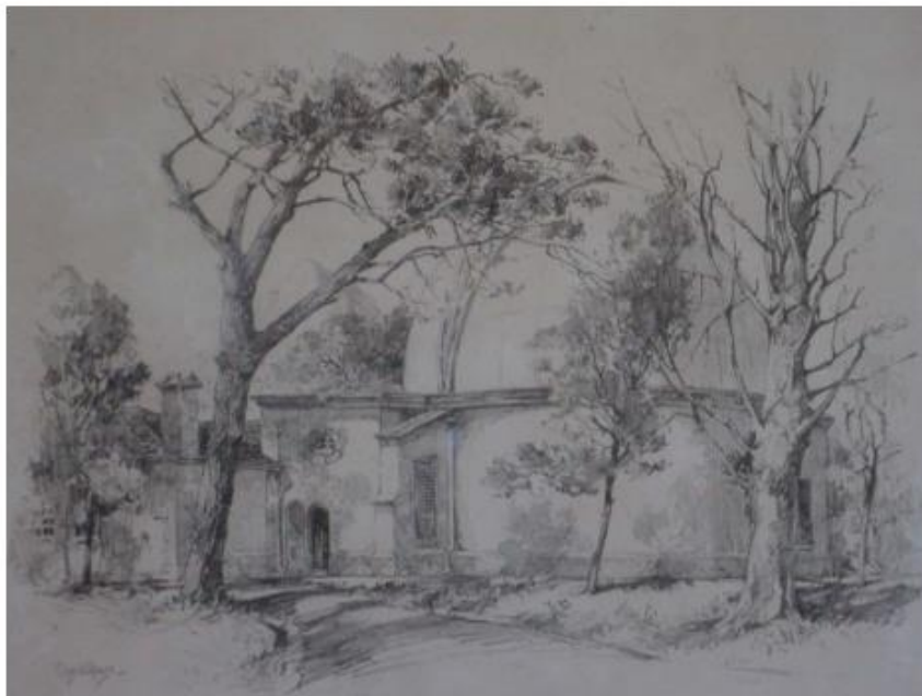
FIGURE 11: Lithograph of the McClean dome, a Herbert Baker building, by artist and astronomer Charles E. Peers (ca 1930) (Ian Glass)
