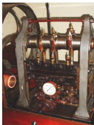
Original hydraulic pump still in use for driving rising floor
