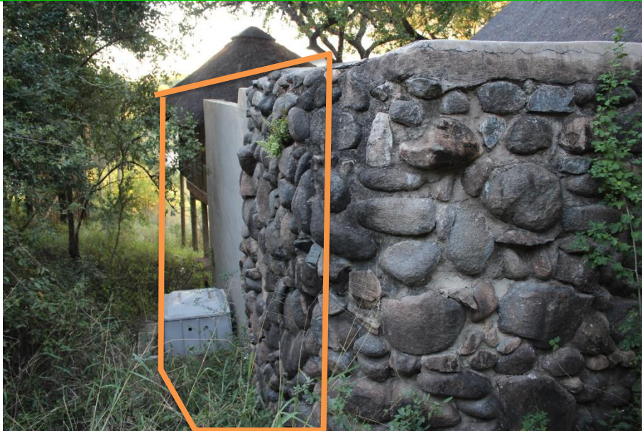
Figure 17: Room 7 new bathroom extension
