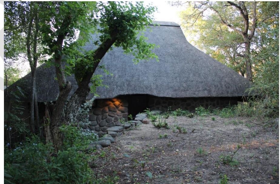
Figure 20: Portion of Room 7's retaining wall to be removed for new access.
