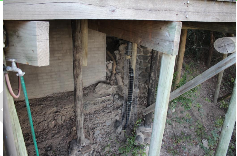
Figure 18: Underneath the deck of Room 7, showing existing footprint
