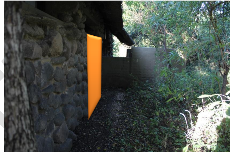
Figure 10: Back of Room 10, showing position of new entrance
