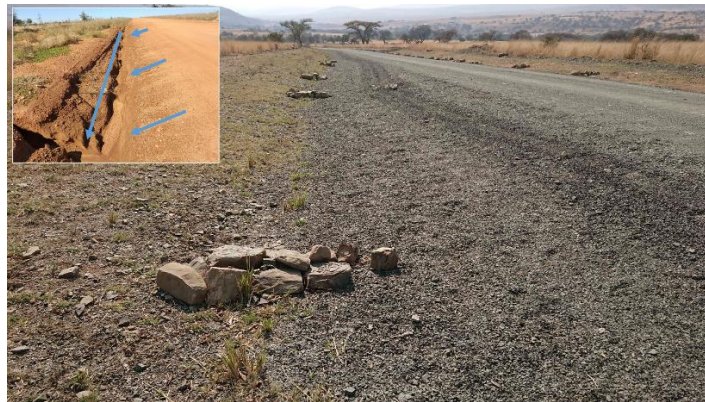
Figure 7-3 Example of road margin erosion prevention
