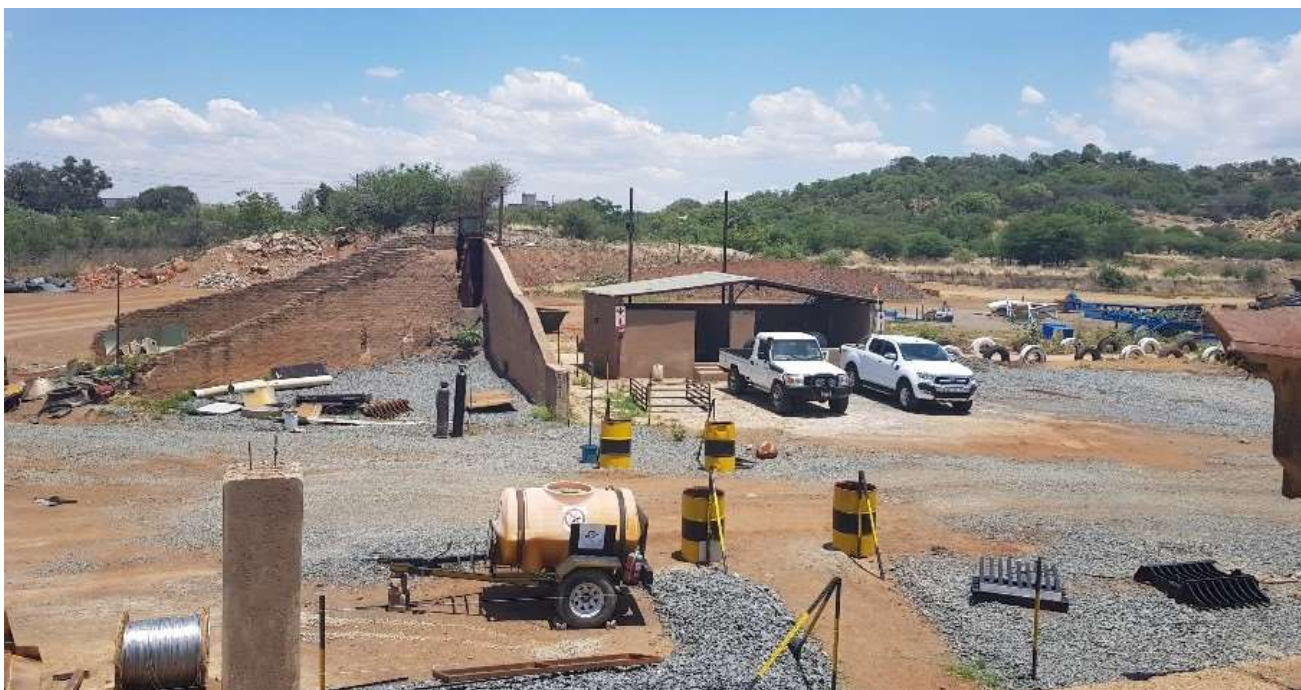
Figure 10-1: Alternative to using water as dust suppression, gravel was put on areas to reduce dust
