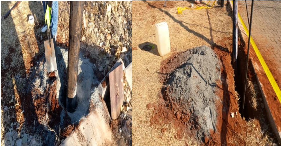
Preparation of Dry mix
