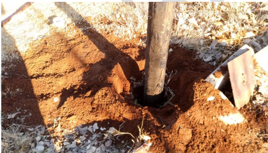
Pole in hole – before backfilling.
