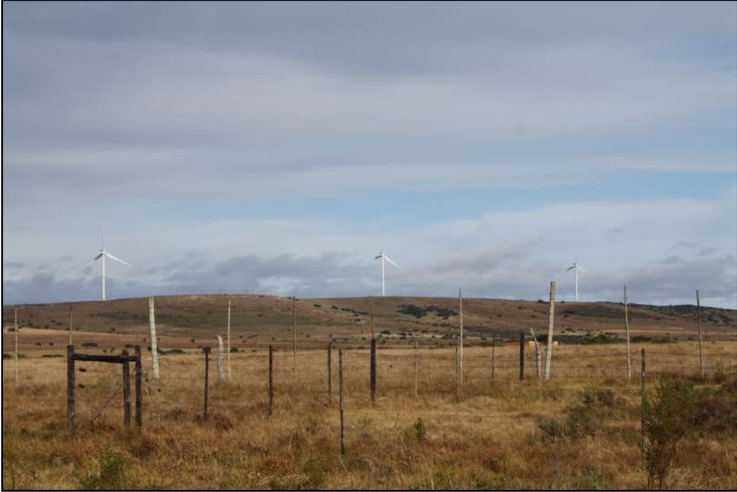
Figure 4: Wind turbines at the Waainek WEF.
