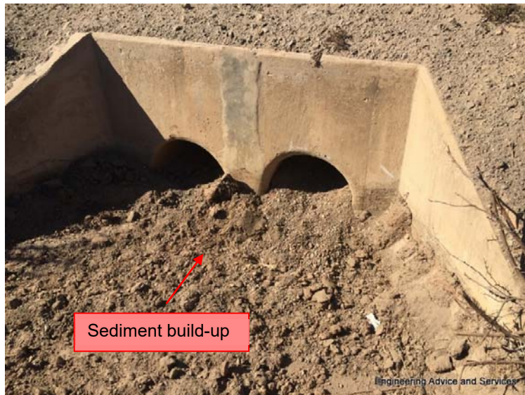
Figure 4 – Typical Stormwater crossing along MR00480
