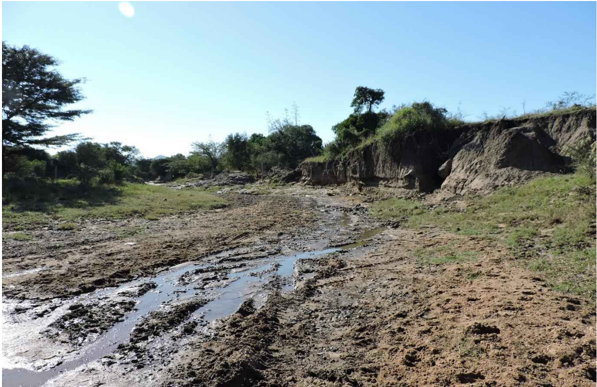
Figure A9: Bank erosion due to a poor vegetation cover.
