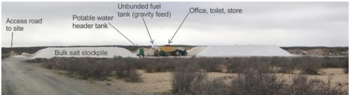
Photo 4: The logistical facility and bulk stockpiling area as viewed from the pan in the south.
