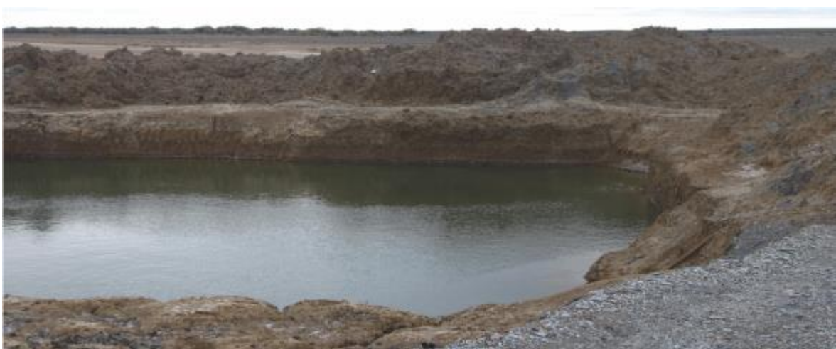
Photo 1: One of the two concentration ponds excavated into the pans into which the brine concentrates. The brine is pumped from here into the evaporation ponds.
