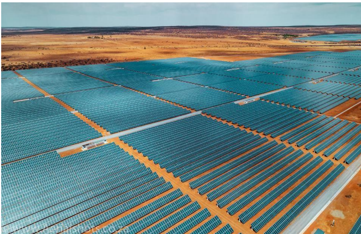
Plate 1 Illustration of PV Arrays at Lesedi north solar field
