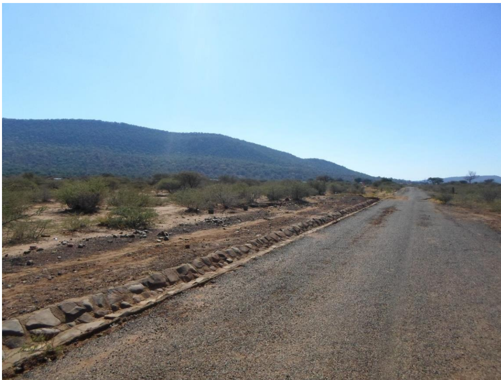
Figure 20: Eastern view from main road through Mantsie towards the proposed alignment
