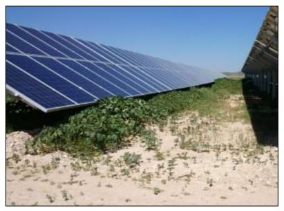
A dense infestation of Stinkblaar (*Datura ferox*) growing at a South African solar PV plant shortly after construction. A large proportion of this invasion could have been avoided if the vegetation beneath the panels had not been cleared as this vegetation would have utilised the water running off the front of the panels and limited the invasion of the *Datura*.
