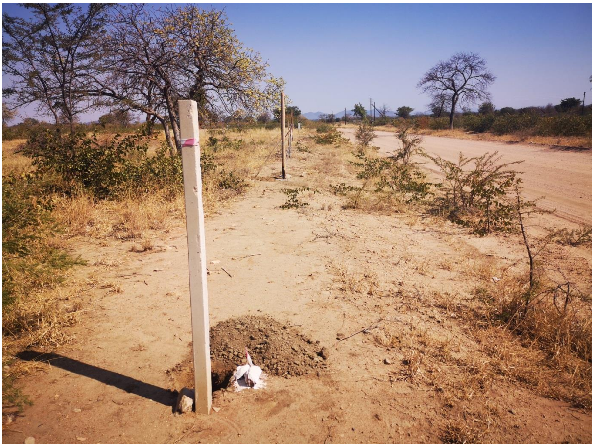
Photo 2: Shows the peg where the powerline is running
