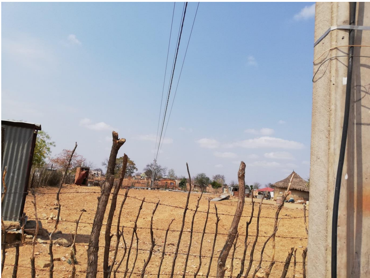
The existing powerline
