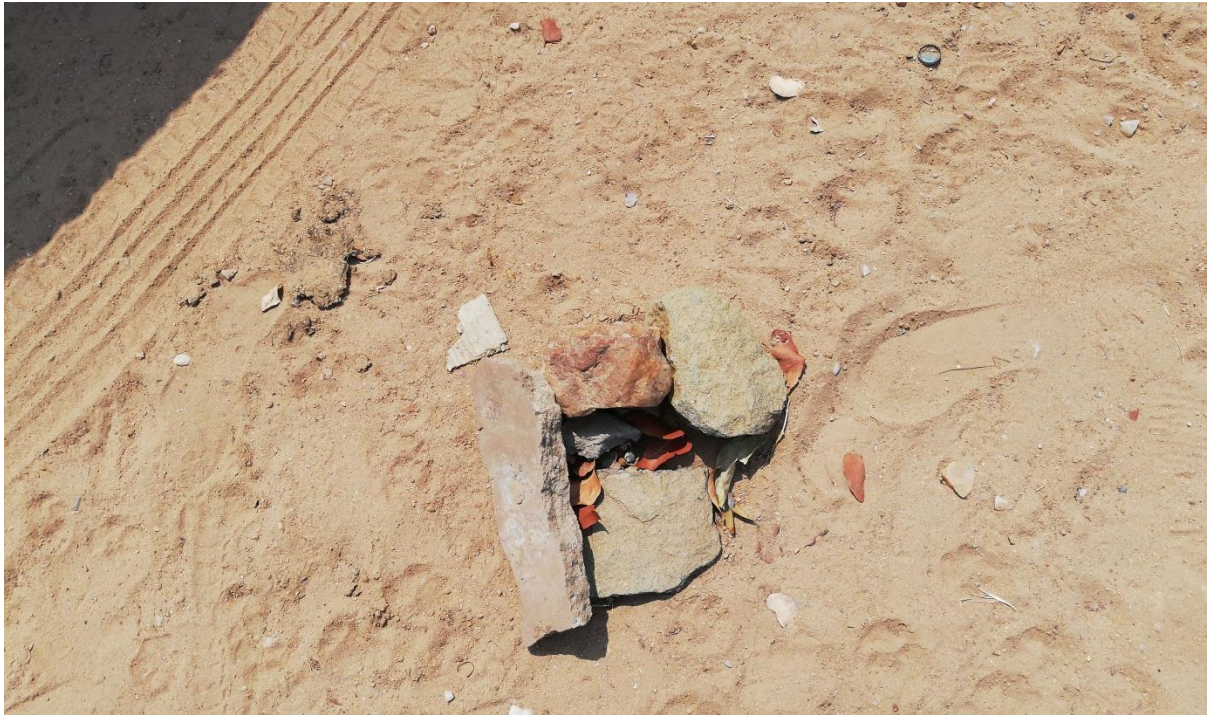
The peg where they are going to plant the pole
