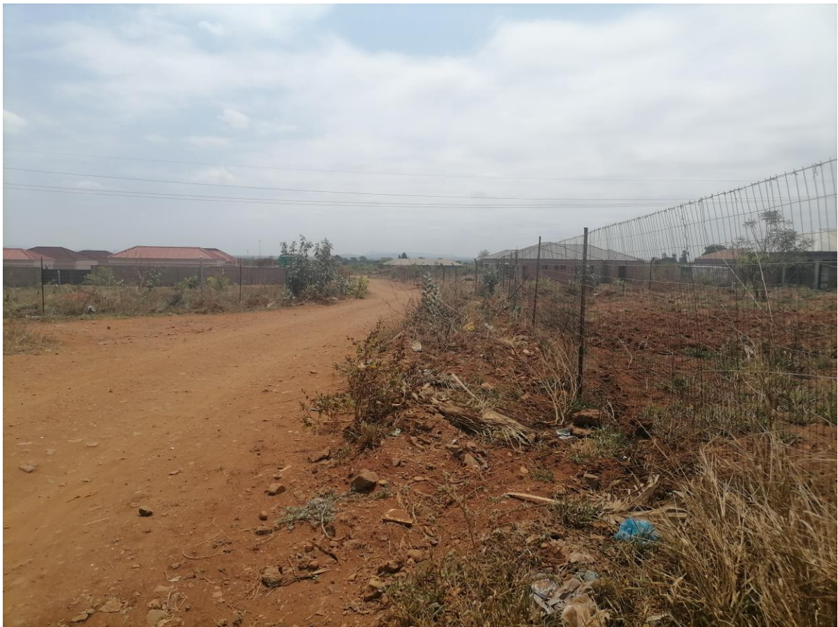
Photo 4: Showing the existing gravel road and the new powerline will be running along the fence
