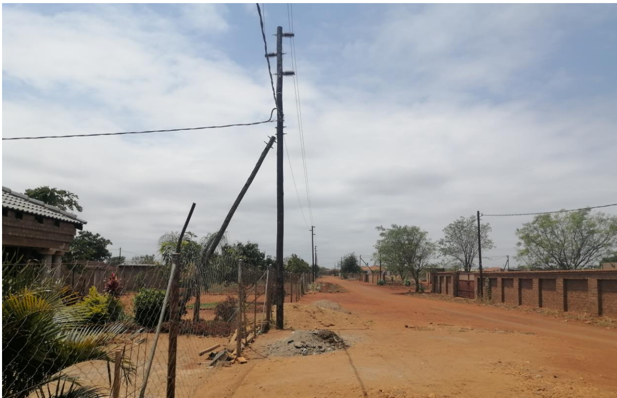
Photo 2: Existing powerline on site
