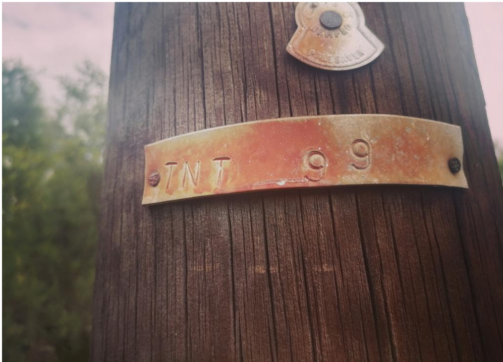
The existing pole number on site, where the line will T-off.
