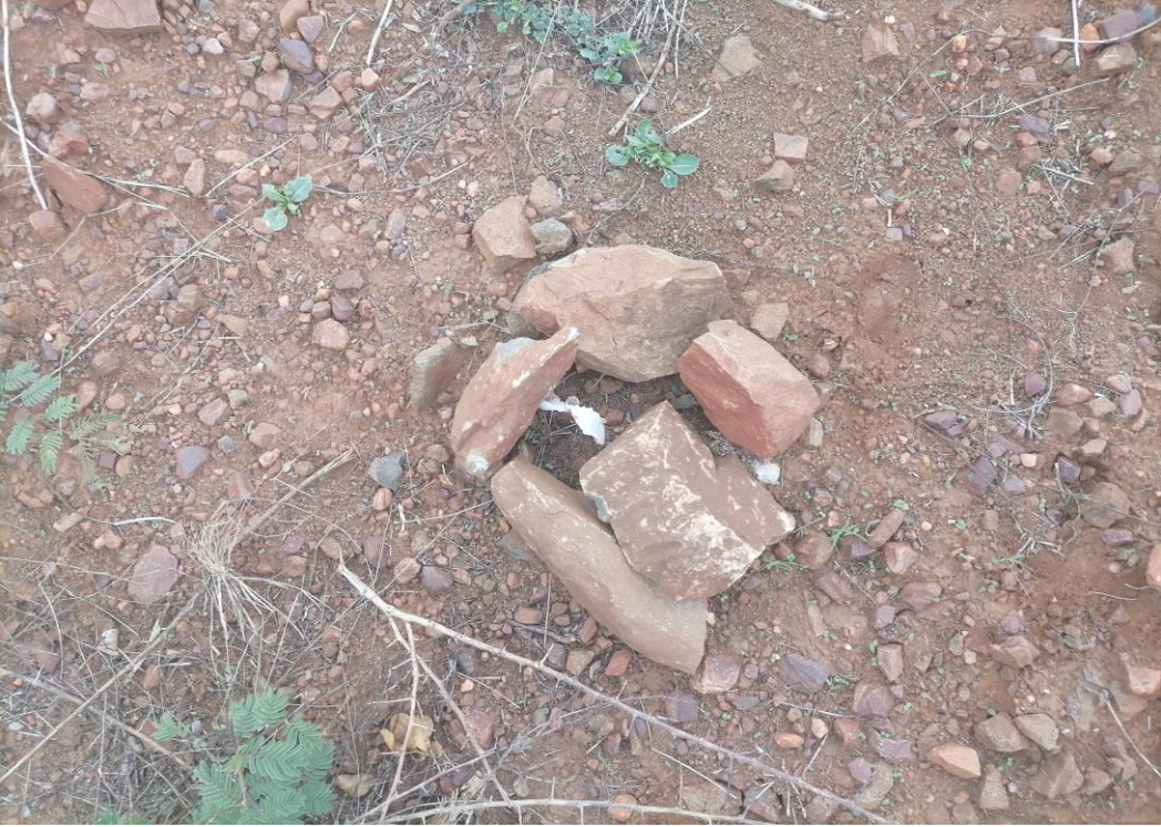
The peg on site where the pole will be planted
