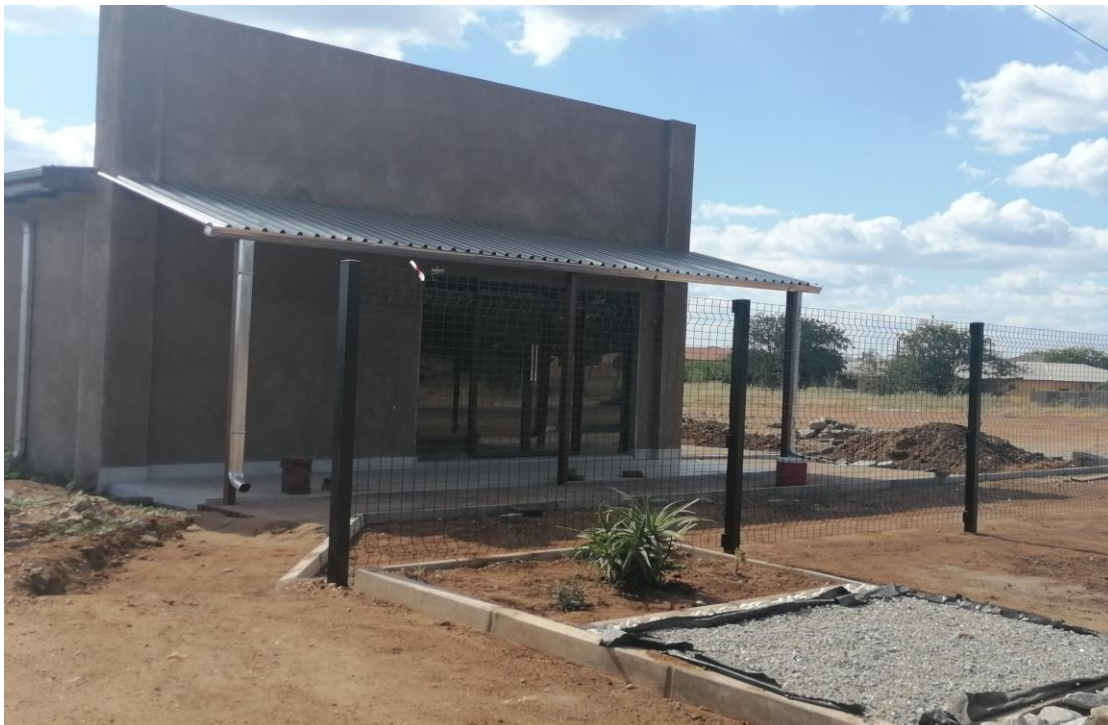
Picture showing the place where electricity supply is needed
