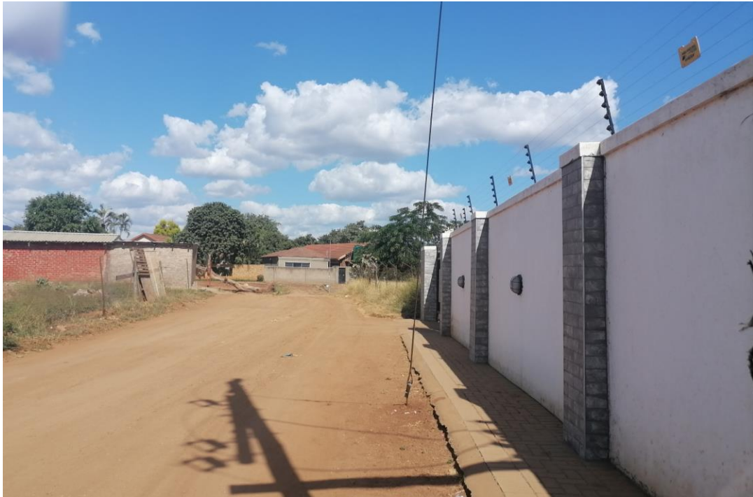
Picture showing the existing gravel road and existing houses
