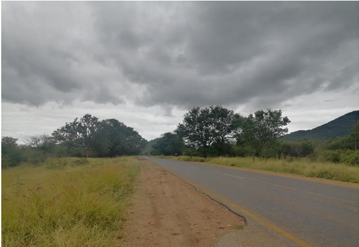
Picture showing the existing tar road
