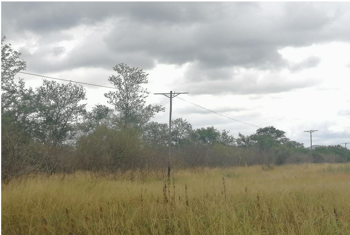
Picture showing the existing Telkom line
