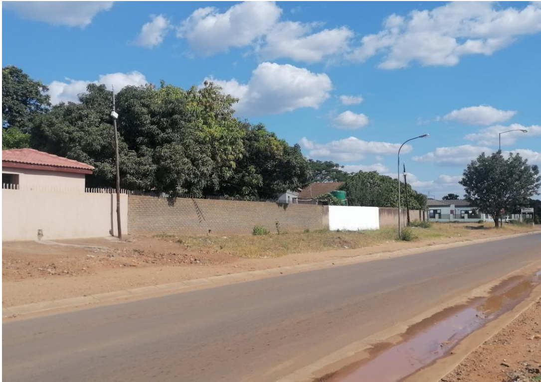
Picture showing the existing tar road and existing houses
