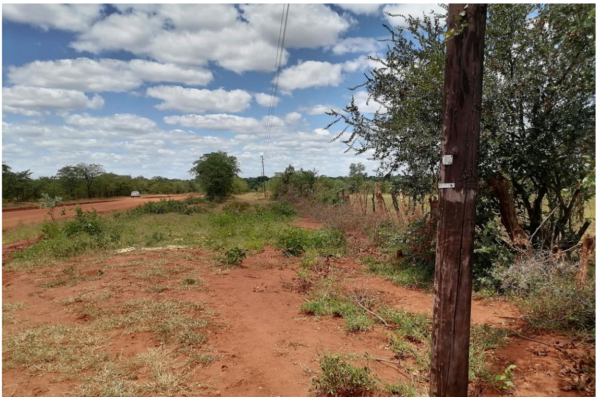
Picture showing the existing Eskom powerline and access gravel road on site
