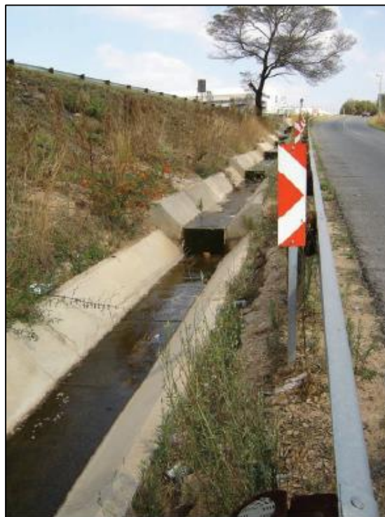
Figure 8: Stepped energy dissipater channel (SANRAL, 2006)
