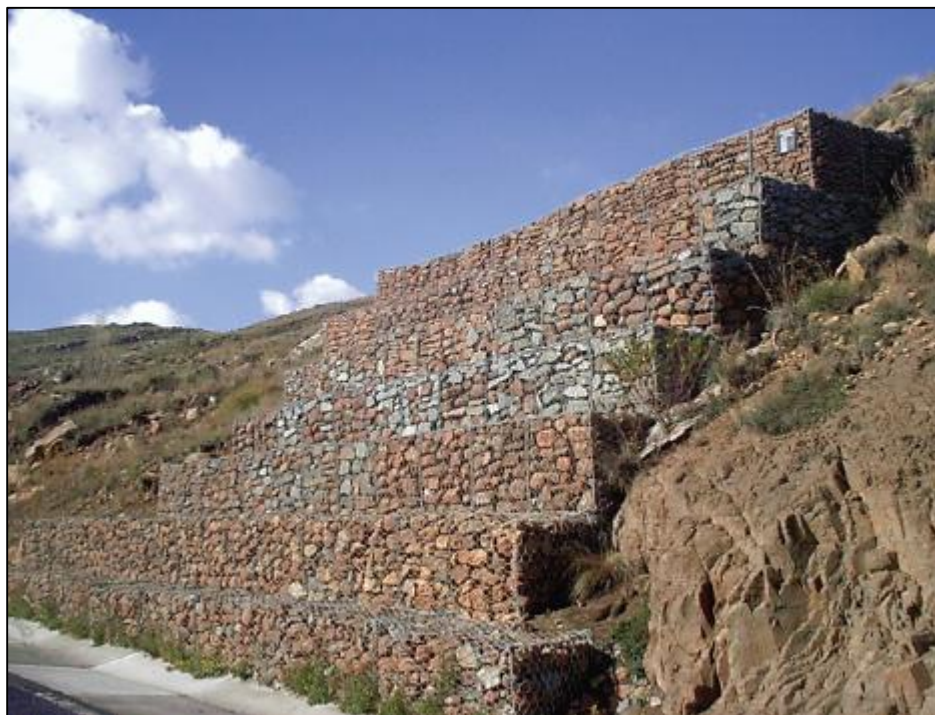
Figure 10: Gabions used for bank stabilisers
