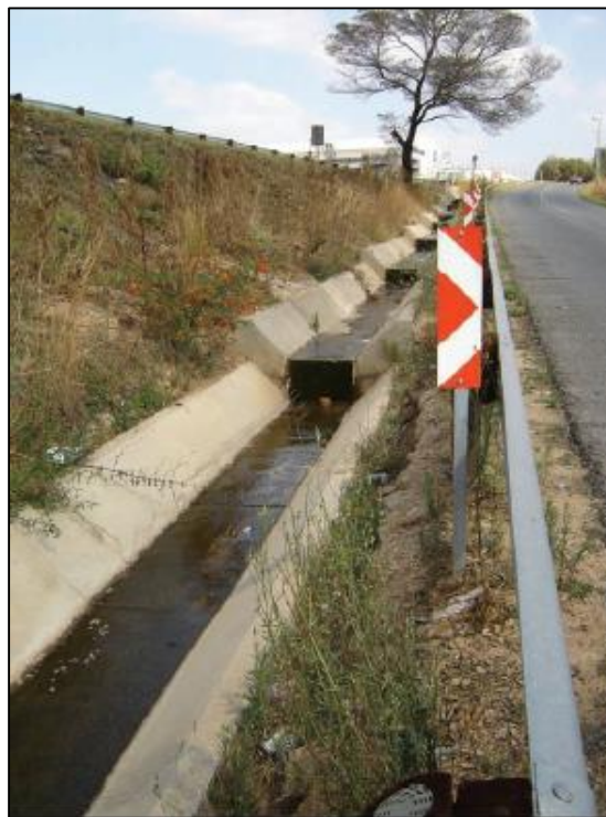
Figure 8: Stepped energy dissipater channel (SANRAL, 2006)
