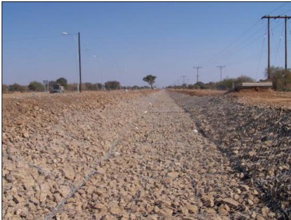
Figure 9: Gabions protection on walls of channel
