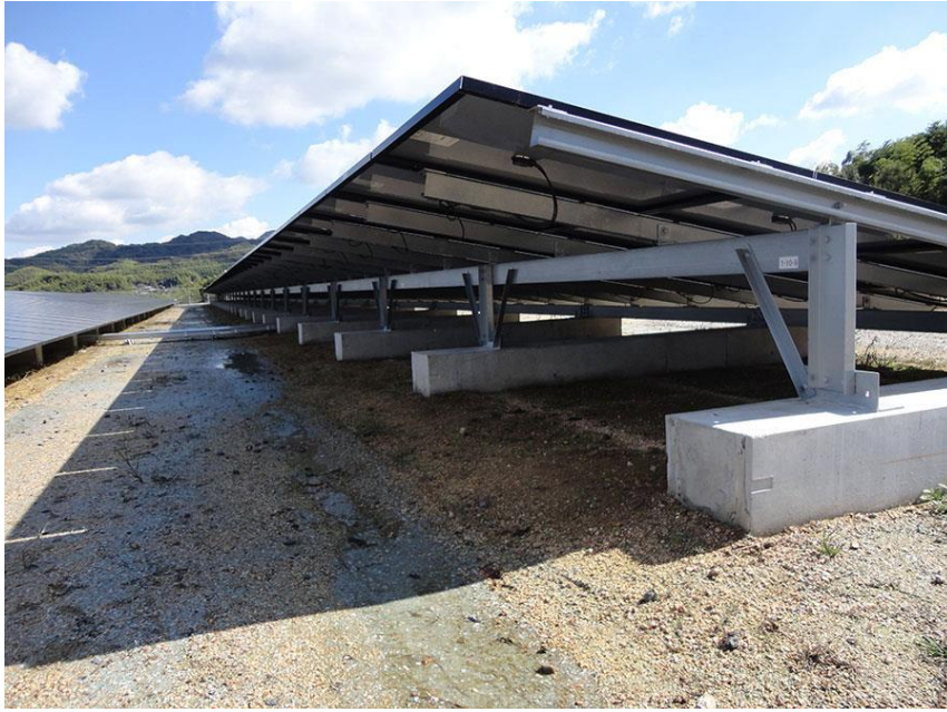
Plate 2: Cast Concrete Foundation (Solar Power Plant Business, 2013)
