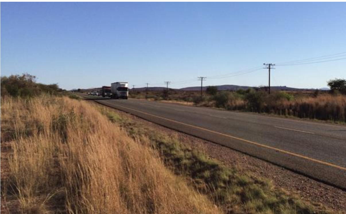
Figure 37: View south from Photo 8 location of the N14 road and the existing telephone lines to the west of the road.
