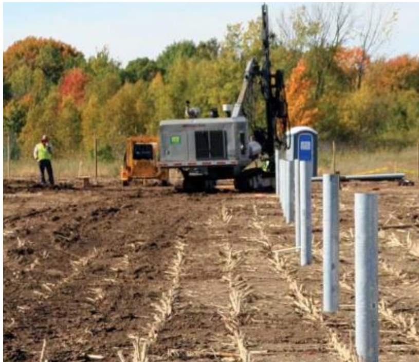
Plate 3: Rammed / Driven Steel Pile (SolarPro, 2010)
