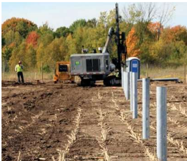
Figure 8: Rammed / Driven Steel Pile (SolarPro, 2010)
