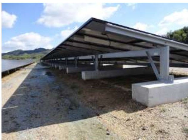
Figure 7: Cast Concrete Foundation (Solar Power Plant Business, 2013)
