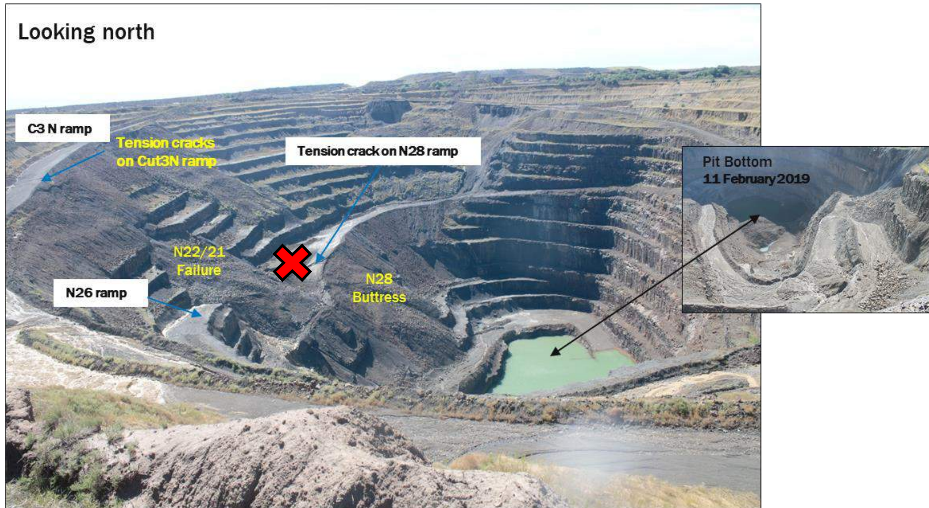
Figure 11. Current status of the open mine pit, looking north, indicating the ramp failures and tension cracks, as well as the forming of the pit lake at the bottom of the pit. Due to the N22/21 and N28 Ramp Failures, the pit is now permanently inaccessible below bench 12, marked with a red cross.
