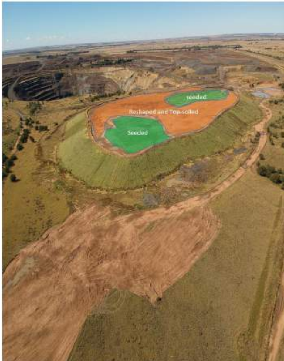
Figure 2. Current rehabilitation of the waste rock dump showing how the mine residue deposits will be reshaped, covered with topsoil and revegetated.
