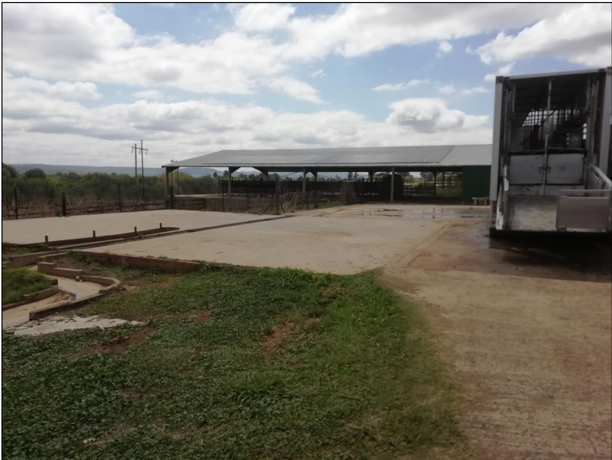
Plate 2: The existing warehouse proposed to house the Rendering Facility machinery. The warehouse already has solar panels installed on the roof.
