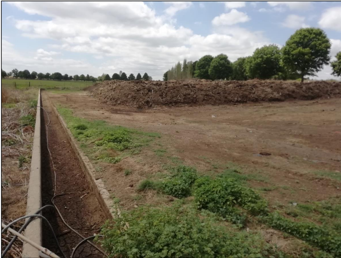
Plate 5: The concrete bunded drain below the Composting Facility which captures runoff from the compost windrows and attenuates it within the bunded catchpit at the end of the drain extent. Water from the catchpit is re-irrigated back onto the composting windrows.
