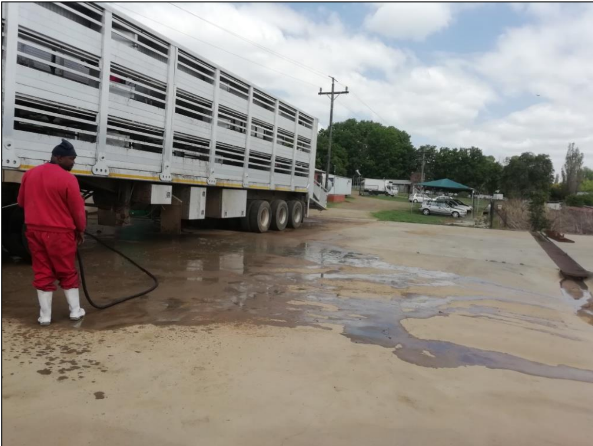
Plate 7: Wash water from washing of piggery delivery trucks is directed towards and captured in a well maintained separated 'dirty water' drain which transfers wastewater directly to the slurry dams. All surfaces are concreted and have a gradient which diverts runoff to the drain and not towards bare soil.
