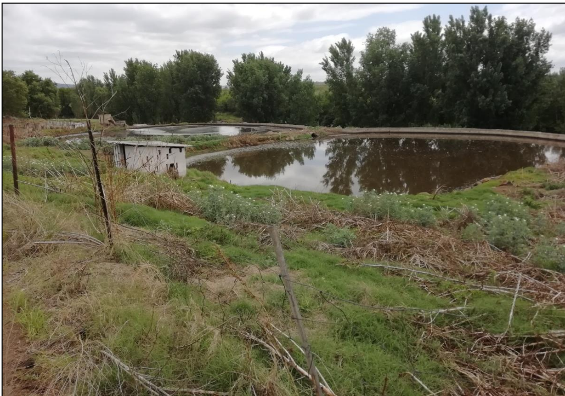
Plate 6: The two (2) existing slurry dams on site which receive wastewater from the abattoir operations and will receive a very small volume of wastewater from the proposed Rendering Facility.
