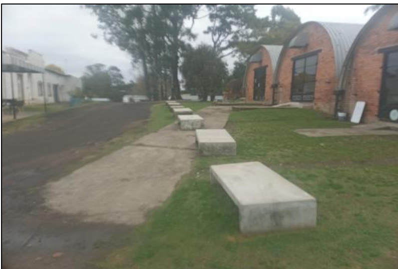
Plate 3: View of the existing shop and retail area.
