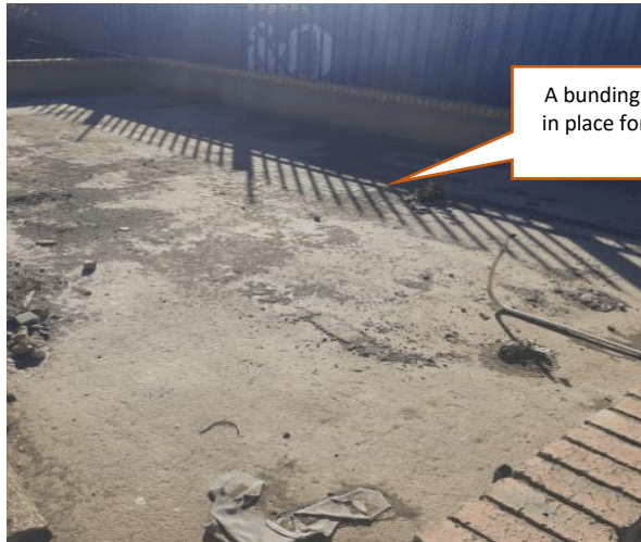
Bunding area for fuel storage already in place. Needs to be signed off for impermeability and capacity.
