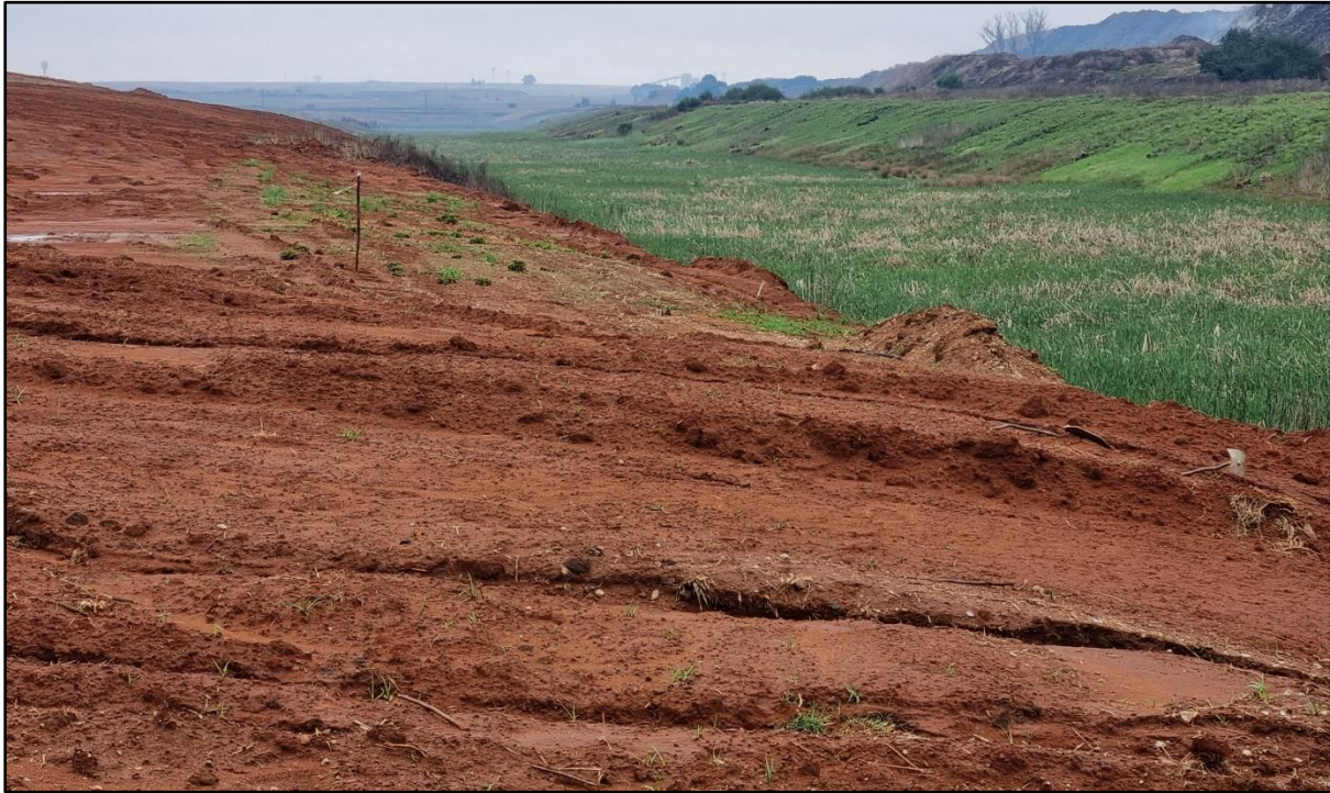
Photo 1: Westward view of the stream diversion channel over the central underground block.
