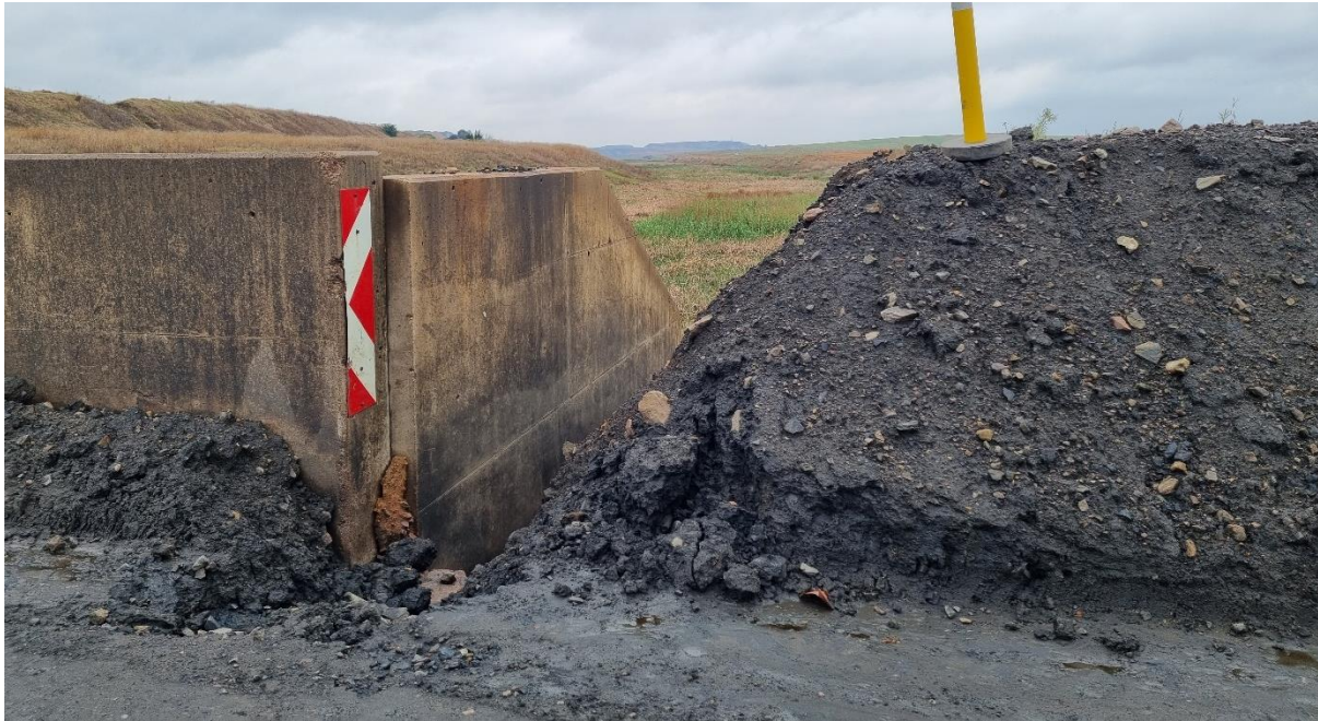
Photo 2: Area where stormwater run-off from the road is allowed to enter the drainage.
