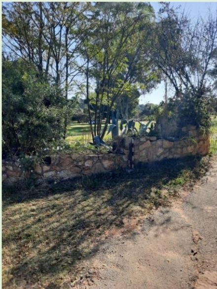
Figure 9: Stone built wall (GH002)
